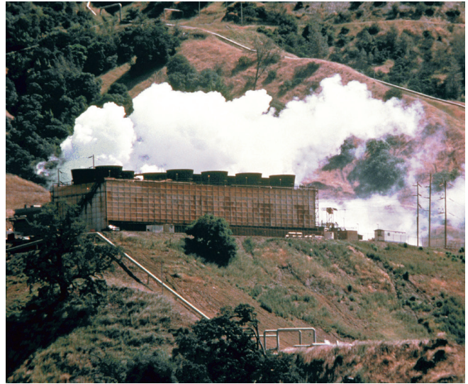
The Geysers, the world's largest geothermal power plant, is in a volcanic area in northern California USGS
