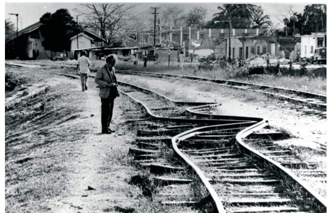
People in the country of Guatemala stand amazed by God's power at a strike-slip fault that moved a ditch several feet! USGS
